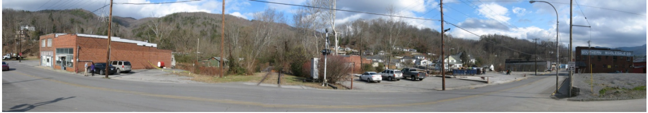
TRAILHEAD B - VIEWING NORTHEAST AT THE RAILROAD TRACKS
